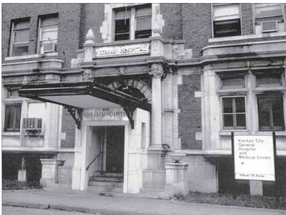
Fig. 8. Before its demolition in 1977, this was an entrance to German Hospital and the subsequent Research Hospital. (Reproduced with permission from Hospital Hill. An Illustrated Account of Public Healthcare Institutions in Kansas City, Missouri . Kansas City: Truman Medical Center Charitable Foundation, 1995, pg. 133.)
